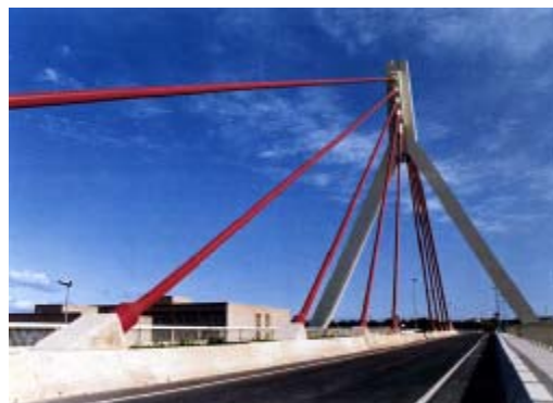
Cable-stayed bridge access to the Technology Park of Valencia. Paterna
